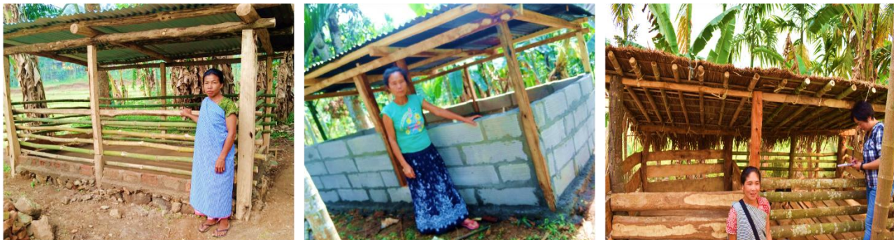
Fig. 2: Representative pictures of the women participants with their pig housing structure during the on-site visit to assess the existing or new housing for pig. Various locally accessible materials like bamboo, wood, bricks, and concrete blocks were used for pig housing.
